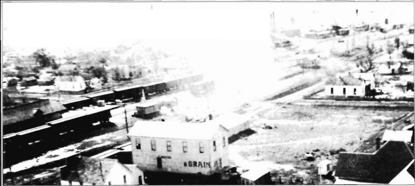
A cameraman in a low flying airplane took this photo of the rail yard and businesses south of downtown Bartlett about 1920. The BW depot is the white building with the words GRAIN written on it. Two BW cars sit on the track beside the depot. The M-K-T depot is across the tracks from the BW headquarters. The cattle pens and several cotton gins can be seen at the upper right.
