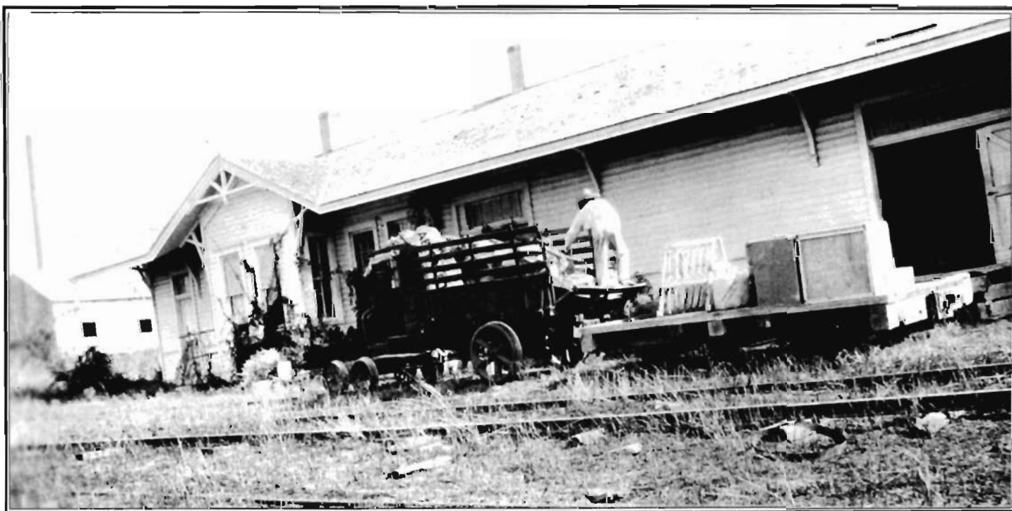
A number of disastrous floods in the early 1920's weakened all the trestles on the BW. The BW locomotives were too heavy to use on the line so alternative power and freight cars had to be built. Cal Breedon, engineer for the company's model "T" Ford, unloads mail and freight at the Bartlett Western depot in Jarrell, Texas. Part of the Harvell cotton gin can be seen at the left north of the depot.
